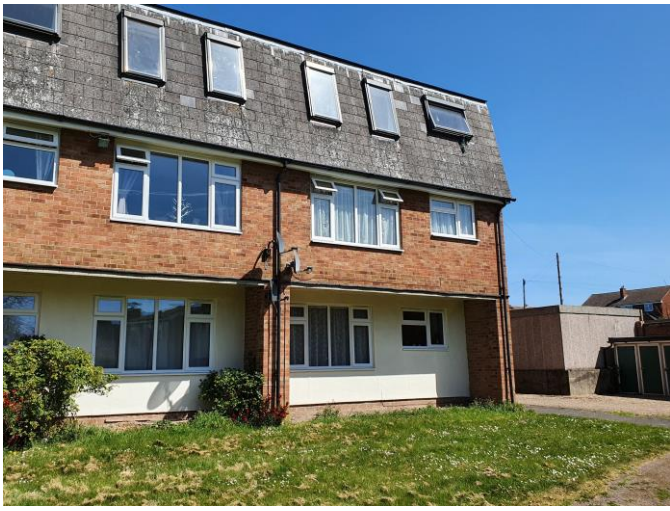
Rear view of block
